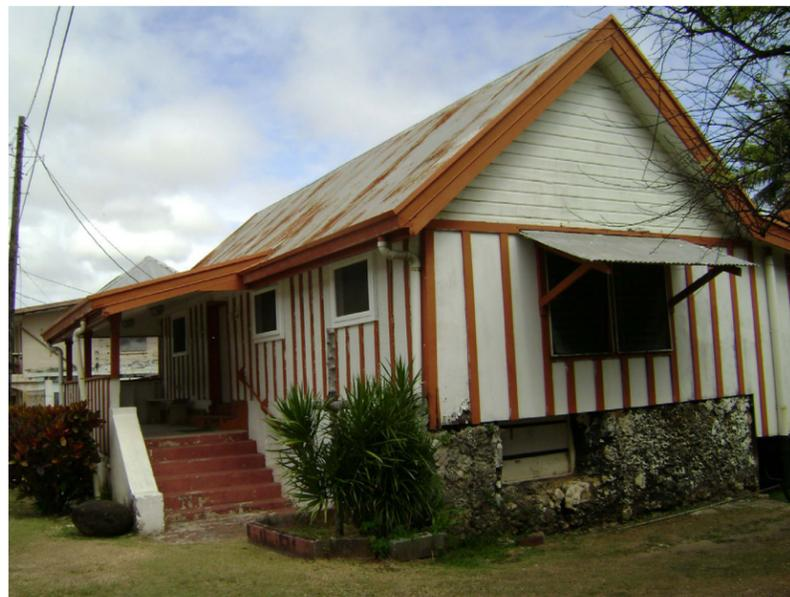
Example of sloped roof, massive exterior stairs, bead board siding, and mamposteria bodega
